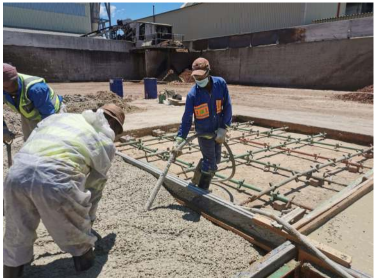
Concrete Leveling in Re-enforcements
