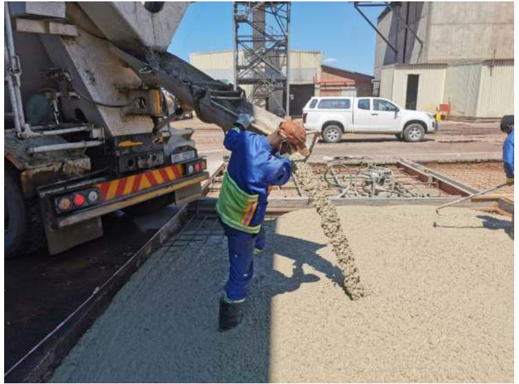
Concrete Leveling in Re-enforcements
