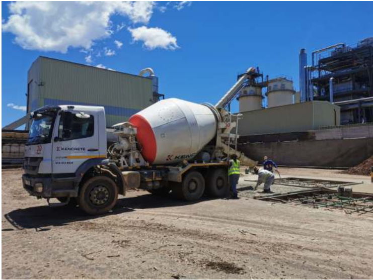
Concrete Leveling in Re-enforcements
